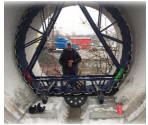
Packer for pipe 96" pipe with cunette
