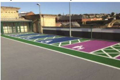
Exposed Deck & Ramps
