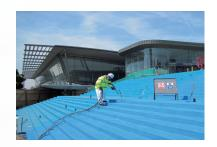
Protection to vertical, sloping and horizontal surfaces to give a fully bonded waterproofing layer to features such as stairs.
