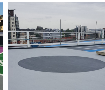
Ramps & Turning Circles
