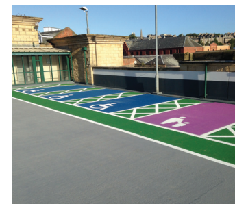
Exposed Decks & Ramps
