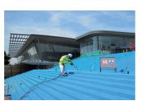
Protection to vertical, sloping and horizontal surfaces to give a fully bonded waterproofing layer to features such as stairs.
