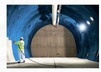
Waterproof layer to the walls and soffits of tunnels and culverts as part of a fully integrated lining system.
