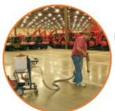
Epoxies and polyureas are used for industrial concrete floor repair and coating.
