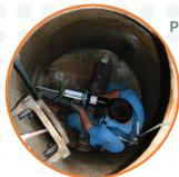
Polyurethane, epoxy, and acrylate injection resins are used for leak sealing and soil stabilization.
