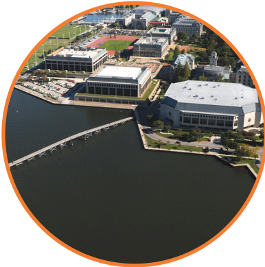
U.S. Naval Academy Seawall
